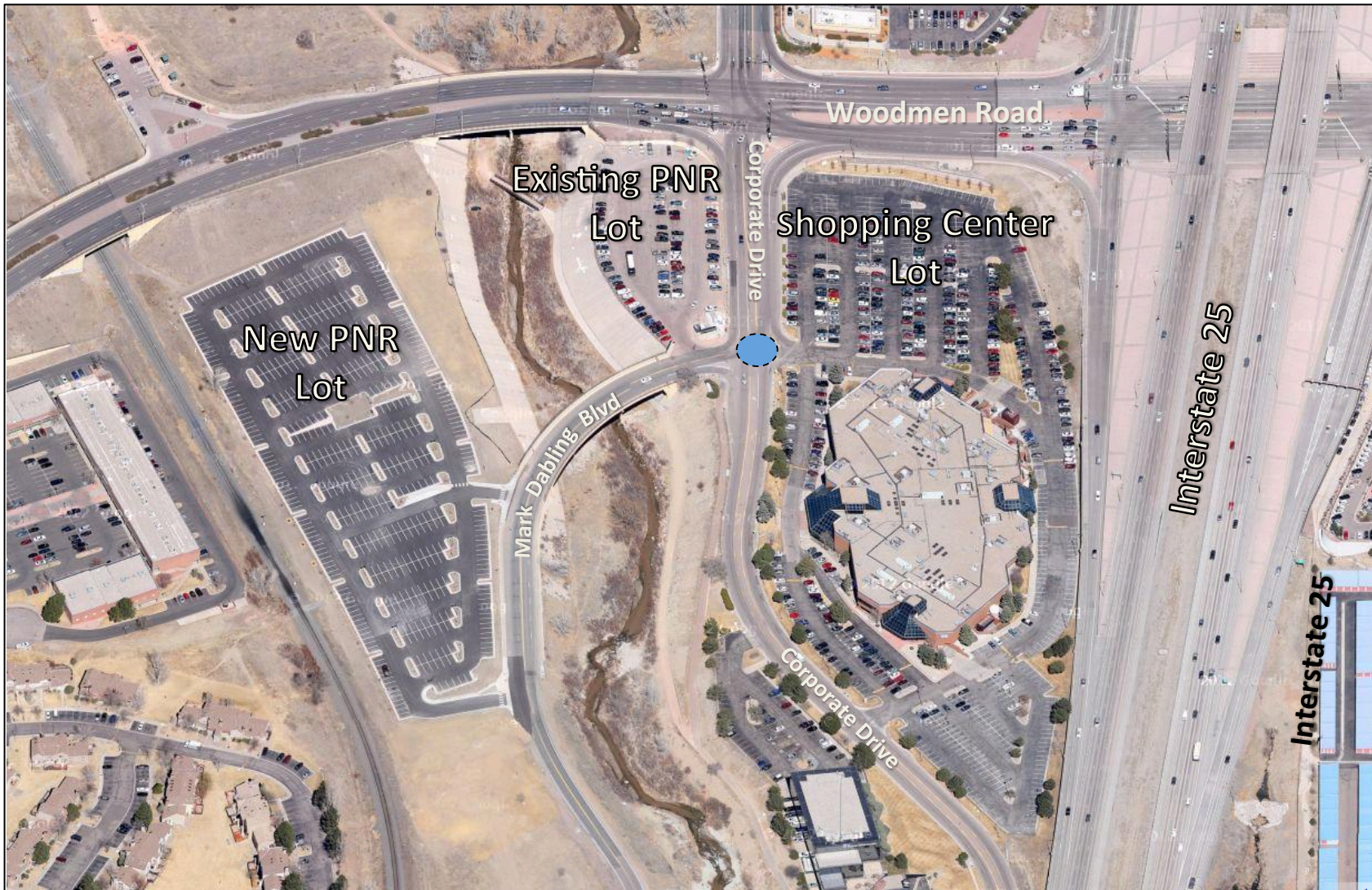
Figure B-2: Site view of Woodmen Park-n-Ride
